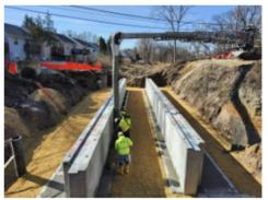
This week, the contractor will be setting up the three-sided structure archways and waterproofing the three-sided structure.
