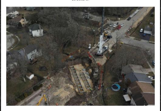
Last week, the contractor utilized a concrete conveyor belt truck to place the concrete for the three-sided structure footings.
